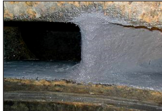
Rebuilt with ARC 858 and ARC 897
