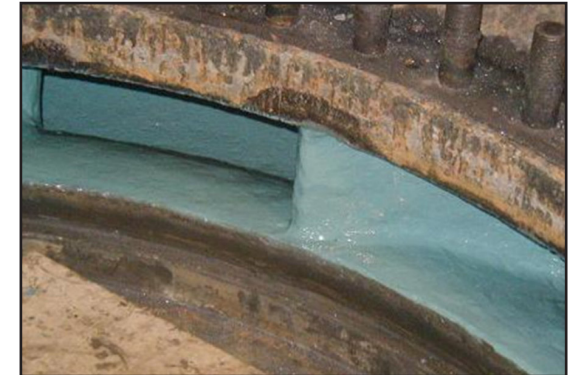
Top coated with 2 coats ARC S2
