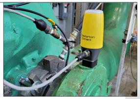
Chesterton Connect sensor connected to split case pump.
