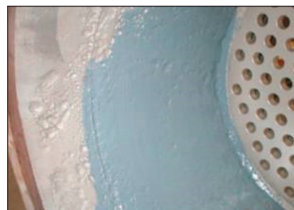
After surface preparation ARC 858 is applied to pitted and corroded areas.
