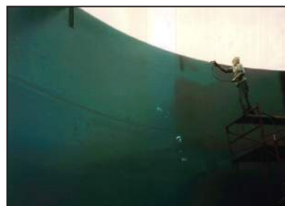
ARC S2 spray applied with airless system
