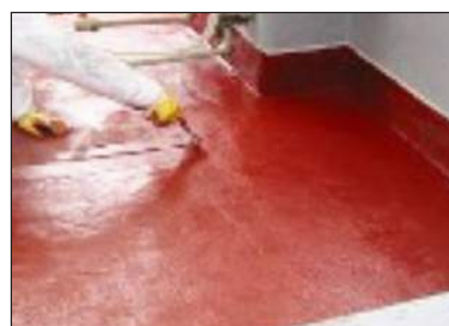
Applying ARC CS4 topcoat to secondary containment.
