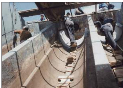
ARC 791 applied to properly prepared surfaces
