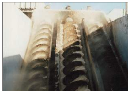
Three effluent pumps in operation prior to repair
