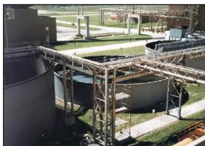
One of four tanks to be lined
