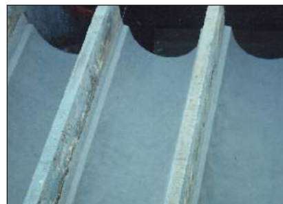
All three pump troughs coated with ARC 791
