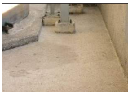
Cleaned and prepared surface of secondary containment.
