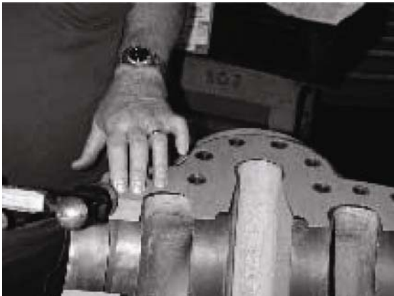
Figure 23: Trimming Casing Gasket
