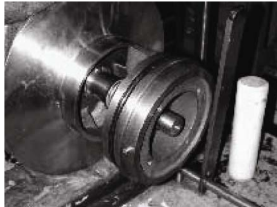
Figure 26: Installing Stuffing Box
