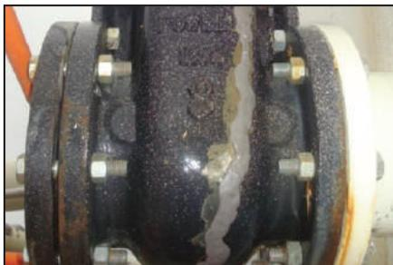
Valve leakage plugged with ARC 5ES.
