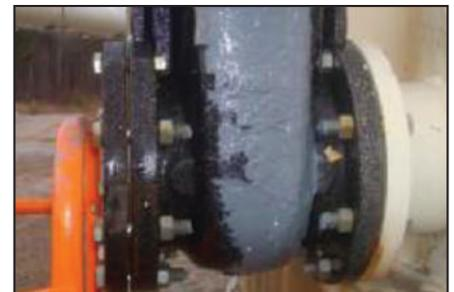
Repaired valve with ARC 5.
