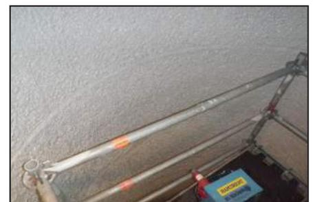
Surface of wet well with final coat of ARC S1HB.
