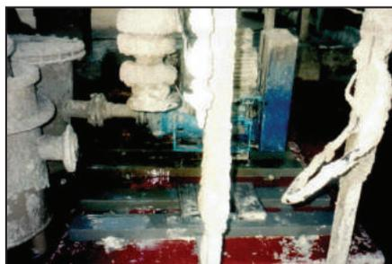
ARC 988 coated pump base: good condition after four years.
