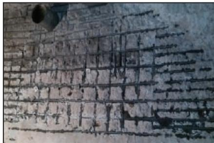
Chest wall after tile removed and blasted.
