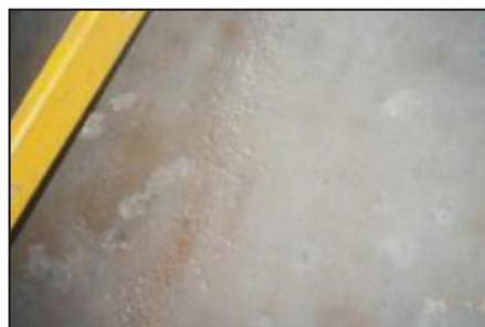
Corrosion and pitting on the spillway gate.
