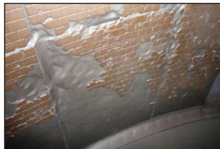
Damaged pulverizer walls.
