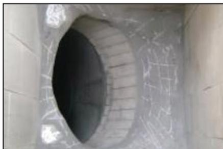
Damage to existing ceramic tiles caused unscheduled shutdown and loss of production.
