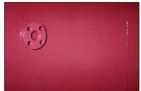
After proper surface preparation, **ARC S4+** was applied in a two-coat system.
