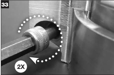
Install new gland cap screws in gland halves.
